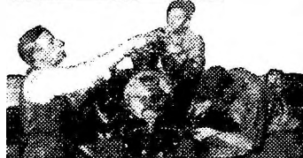
Students wiring and checking ignition on one of the late type Radial Aircraft Engines in our aviation department
